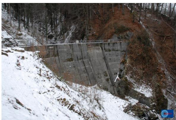
Abb. 3.1a: HRB Schlundbach ( https://ssl.panoramio.com/photo/50363051.jpg )
